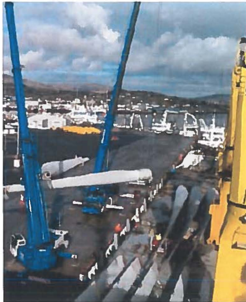
Figure 5. Unloading Turbines at Killybegs. (Source: Killybegs Harbour Centre)
